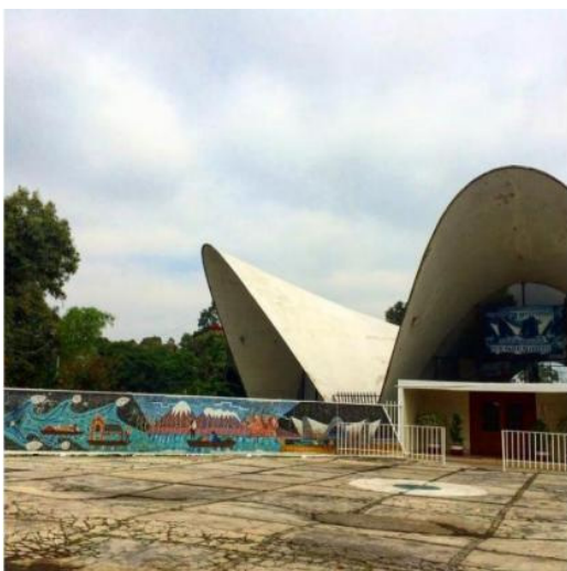
Figure 8. View of the main facade in which the formation of the hyperbolic paraboloids and their continuation of the reinforced concrete shell can be seen
