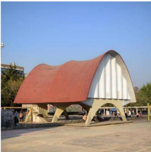
Figure 3. Pabellon de Rayos C6smicos, Felix Candela's first hypar structure
