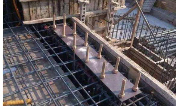
Figure 1 Construction of Roof Reserved Holes
