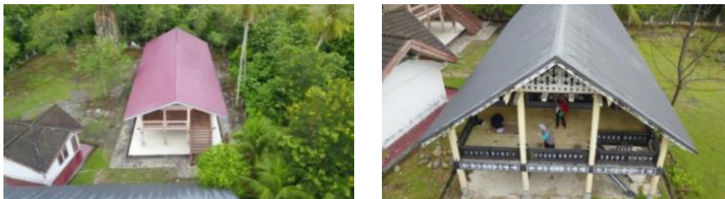
Figure 4. Roof conditions UPR 1 (left) and UPR 2 (right).
