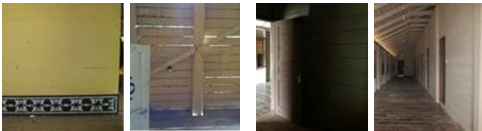
Figure 5. Wall condition of UPR 1 (left) and UPR 2 (right).
