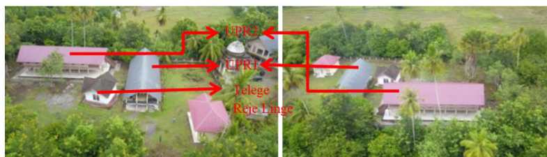
Figure 10. Environmental conditions at the front of UPR 1 and UPR 2.
