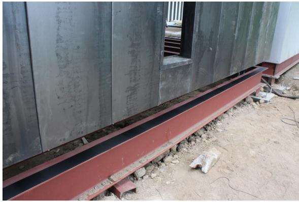
Figure 15. HDPE joint in the support of the panels.
