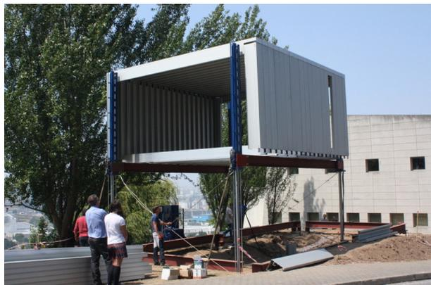
Figure 14. Positioning of the jacks and lifting of the aluminum module with the bracing cables.
