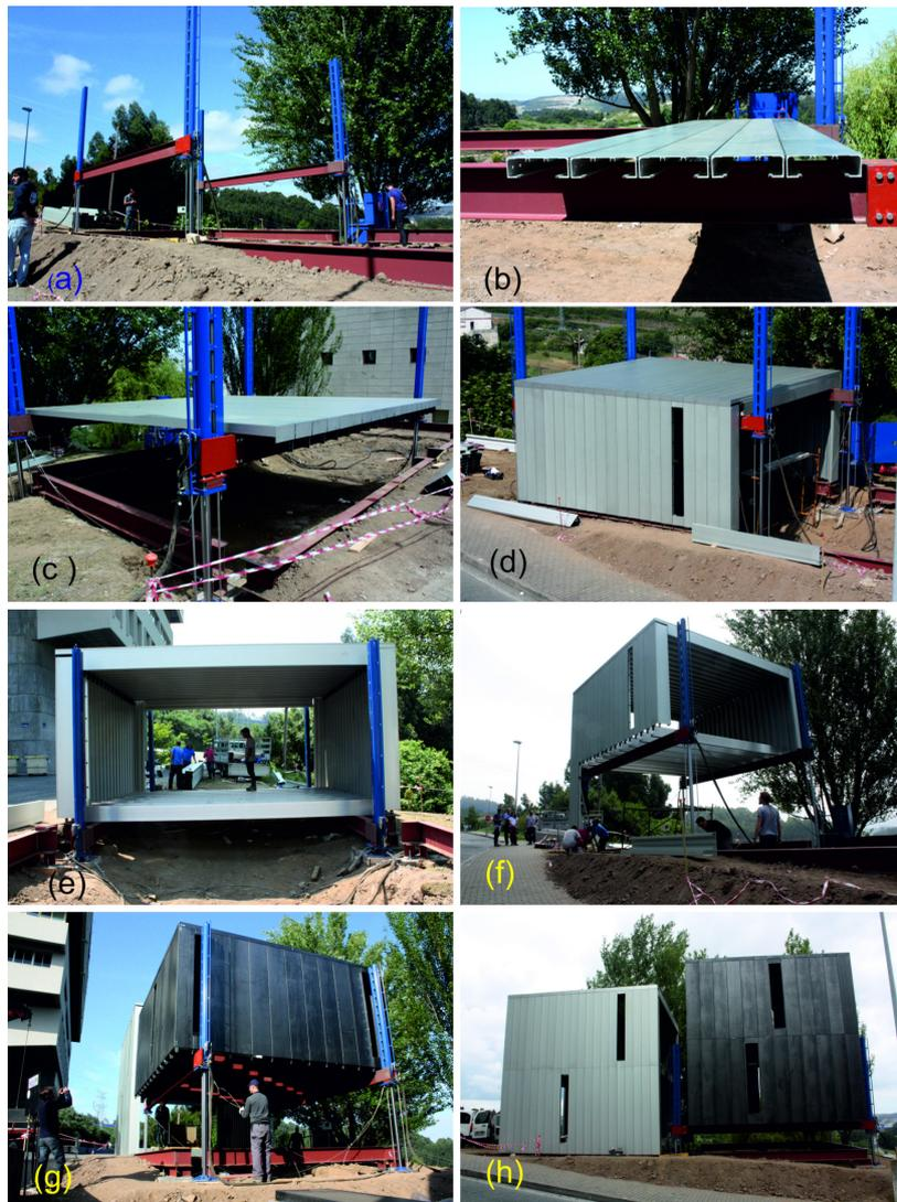
Figure 4. Construction phases of the Reverstop module.
