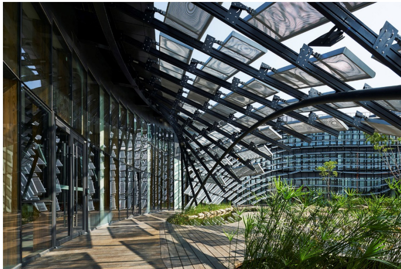
Figure 9. The maximized use of natural lighting and use of shading devices to prevent the glare.
