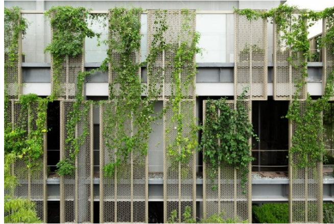
Figure 4. This figure shows the green facades is similar to green walls but integrates with the architectural elements like windows and terraces. [40]
