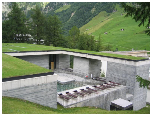
Figure 8. The integration of green elements with the building design especially the green roof.
