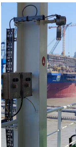
图15 GAS DETECTOR ( WALL MOUNTING )
